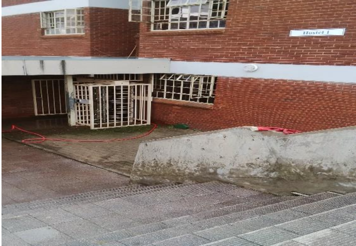
Figure 10: Picture showing an inaccessible door to the hostel
