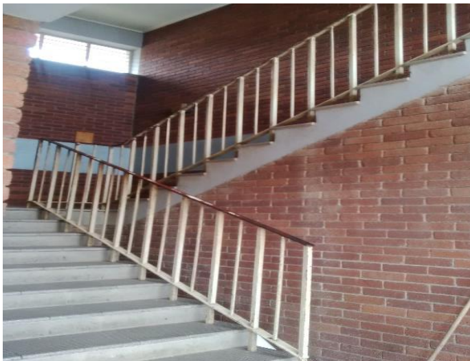
Figure 9 Picture showing an inaccessible lecture room
