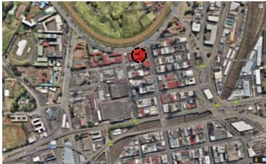
IMAGE 73: Thokoza Female Hostel located on the edge of Greyville racecourse SOURCE: https://www.google.co.za/maps
