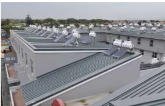
IMAGE 38: Solar panels used to heat water are fitted to the roofs of the units SOURCE: http://www.nhfc.co.za
