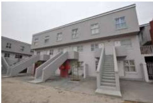
IMAGE 33: The stairs contribute towards social interaction among the resident's and allows first floor units immediate access the ground floor. SOURCE: http://www.nhfc.co.za
