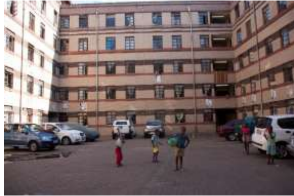
IMAGE 83: children have to play on harsh concrete and brick surfaces within the courtyard spaces. SOURCE: Picture taken by the author
