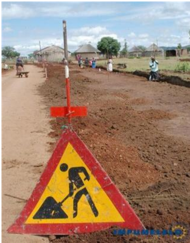
Figure 4.1: Gundo Lashu Road Works
