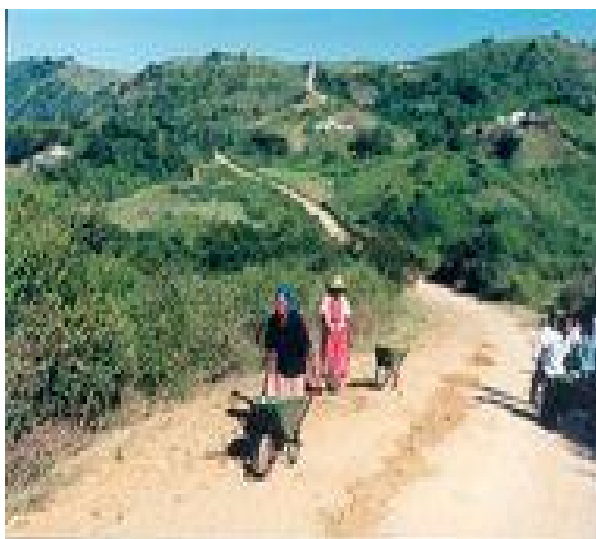
Figure 4.2: Zibambele Road Works
