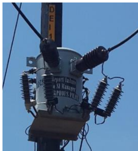
Figure 2 - 5: 16 kVA transformer installed at a pilot site (Courtesy of Eskom)
