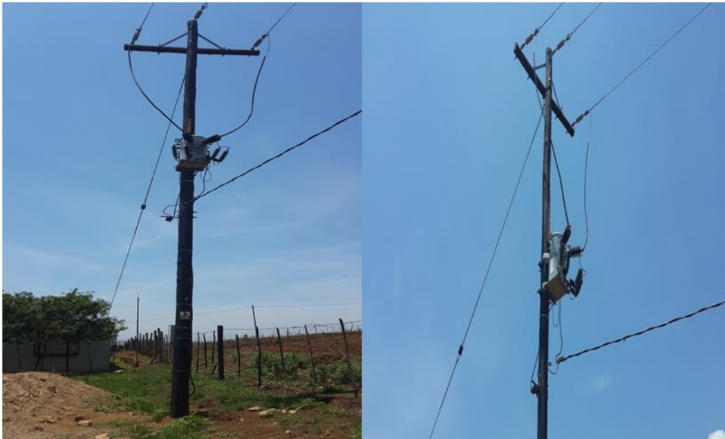
Figure 1 - 1: 16 kVA Transformer installation (courtesy of Eskom)
