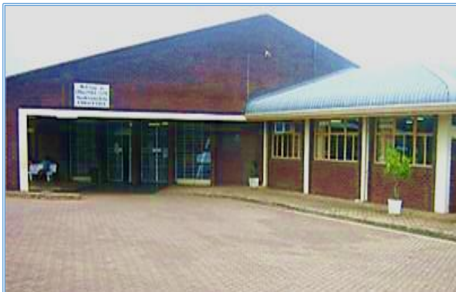
Figure 3.1: Imbalenhle Community Health Centre
