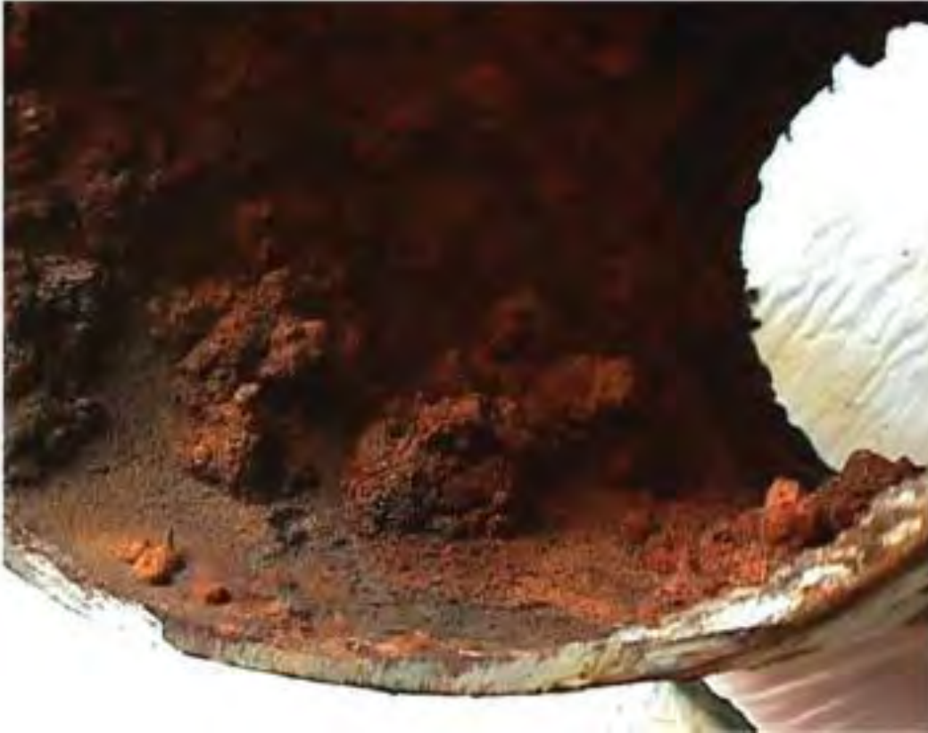
Figure 2.1: Biofilm growth and corrosion by-products on a ductile iron pipe (Simoes & Simoes, 2013).
