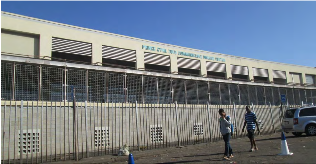
Figure 66: Front facade of building off University Avenue. A fence acts as a barrier and the building elevated from ground level.
