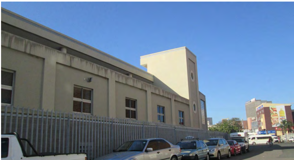
Figure 72: Rear facade of building.
