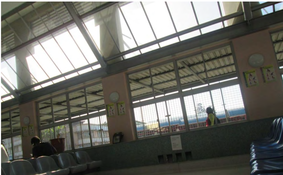
Figure 68: A view to the outside from the TB clinic waiting area
