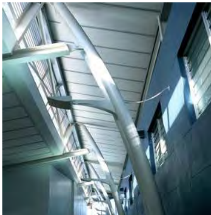
Figure 59: Light and fresh air filters through from the clerestory and vents above.
