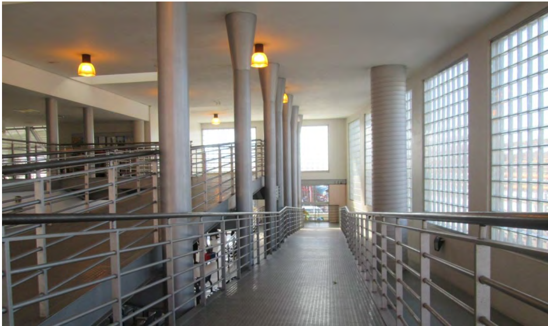
Figure 70: Ramp access to the upper floor and glass bricks along facade to allow maximum natural light.
