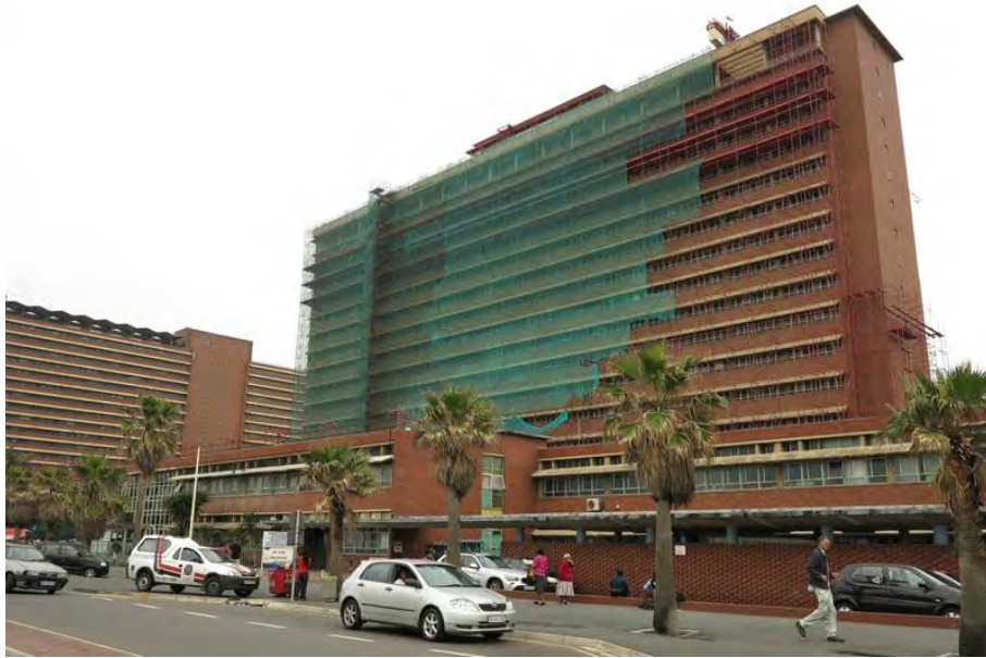
Figure 7: An image depicting Addington Hospital, a state facility situated within Durban CBD, South Africa. This is the general identity of state healthcare facilities in the country.
