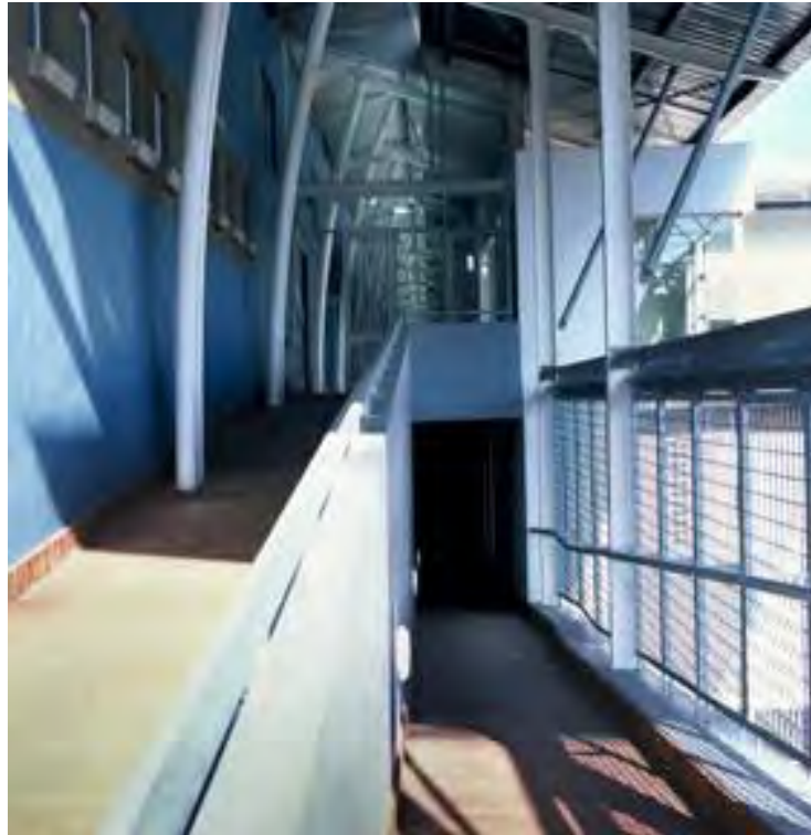
Figure 60: Ramp to the lower ground on the west edge.
