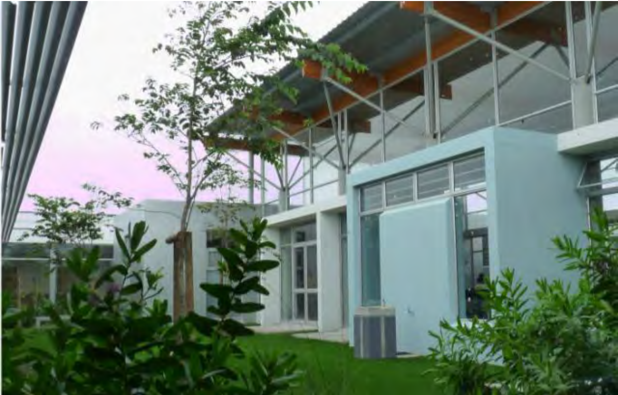
Figure 42: View of the main waiting area from the courtyard.
