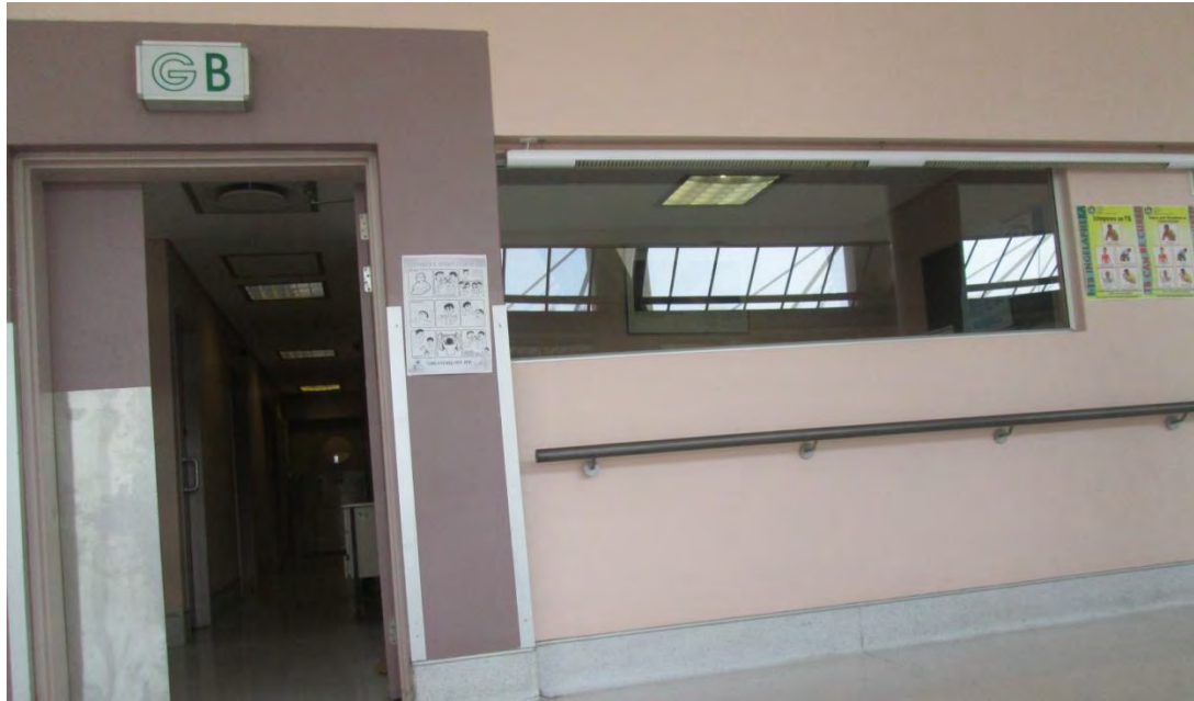
Figure 69: A clinical finish to the institute walls and floors
