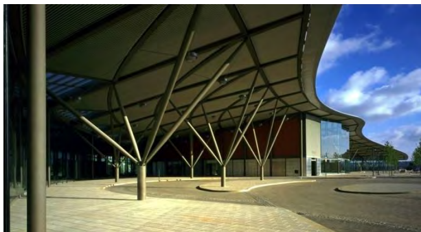
Plate 7.10: shows the curved roof structure of the external concourse (Source: http://www.fosterandpartners.com/projects/north-greenwich-interchange/ 14 May 2014)
