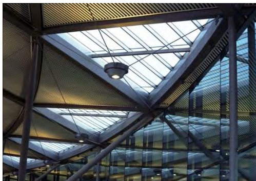
Plate 7.12: Shows the perforated roof sheeting and the specially designed light. (Source: http://www.fosterandpartners.com/projects/north-greenwich-interchange/ 14 May 2014)
