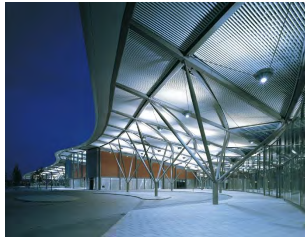
Plate 7.9: shows the general façade of the North Greenwich Interchange (Source: http://www.fosterandpartners.com/projects/north-greenwich-interchange/ 14 May 2014)
