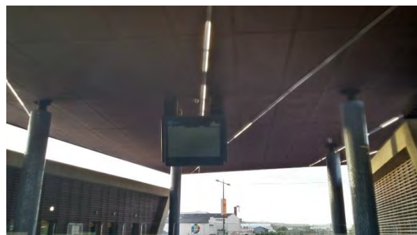
Plate 8.42: Shows the lines continued on the canopy (Source: Author, 2014)
