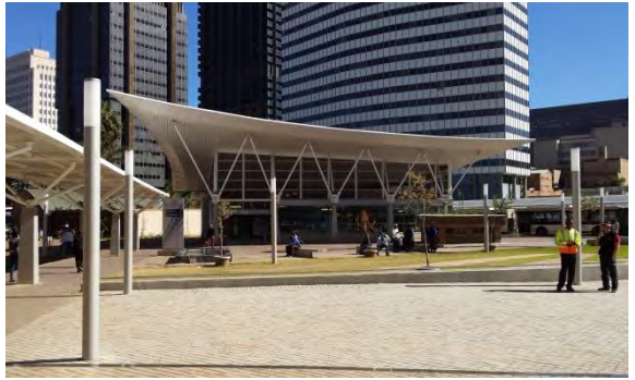
Plate 8.17: Shows the entrance of the newly added Gautrain Station (Source: Author, 2014)
