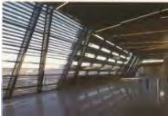
Plate 8.47: Shows how light is conveyed onto the upper level concourse (Source: Peters, 2010: 3)
