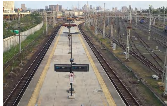
Plate 8.38: Shows train platform waiting areas (Source: Author, 2014)
