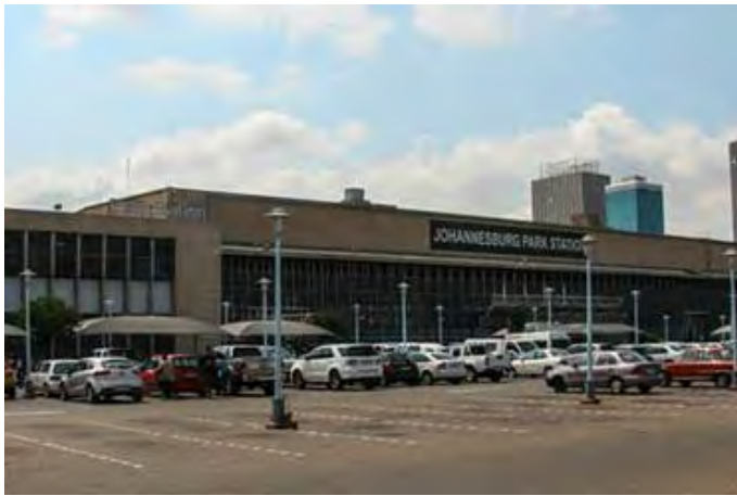
Plate 8.10: Shows Main Station consisting of a brickwork and concrete structure (Source: author, 2014)
