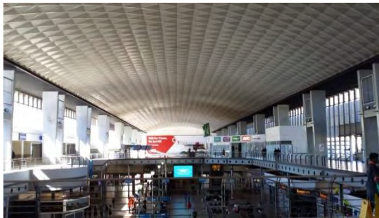
Plate 8.18: Shows the main concourse light weight roof structure and clear storey lighting (Source: Author, 2014)
