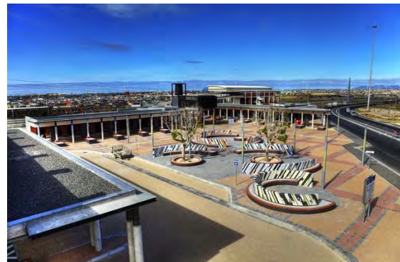
Plate 6.18: shows Kuyasa interchanges connection with the urban realm (Source: http://www.meyervorster.co.za/home.asp?m=7&idkey=542/ accessed 25 April 2014)
