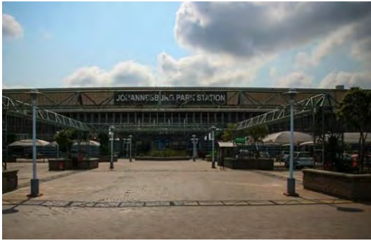
Plate 8.14: Shows the primary entrance of the main station building onto the upper level (Source: Author 2014)
