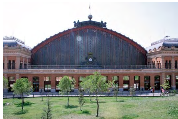
Plate 6.12 shows the symbolic façade fronted by a public square (Source: http://www.landezine.com/index.php/2009/08/botanical-train-station/ - accessed 23 April 2014)
