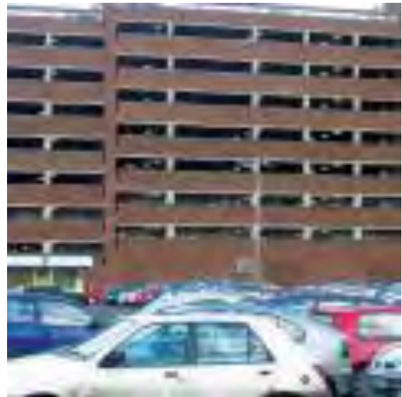
Plate 6.3: Multi-storey carpark in the United Kingdom displays the quality of the current public realm and the built environment. (Source: http://www.rudi.net/node/18505 - accessed 21 April 2014)
