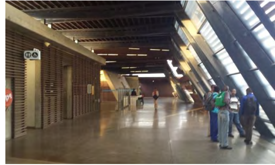
Plate 8.40: Shows canopy structure from the interior concourse (Source: Author, 2014)
