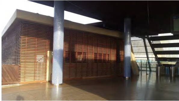
Plate 8.39: Shows the varying canopy structures and the concrete shell form which houses offices (Source: Author, 2014)
