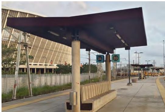
Plate 8.37: Shows the platform waiting area structure (Source: Author, 2014)
