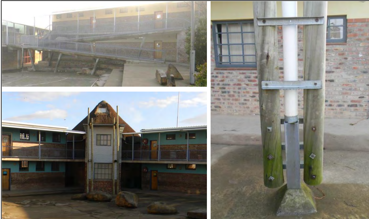
Figure 4.24 (top-left) (Source: Author's Photograph, 2013) : Main ramp system.
