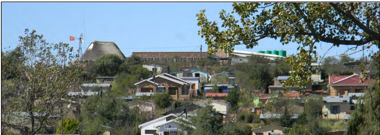
Figure 4.13 (Source: Author's Photograph, 2014) : Building and Surrounding context.
