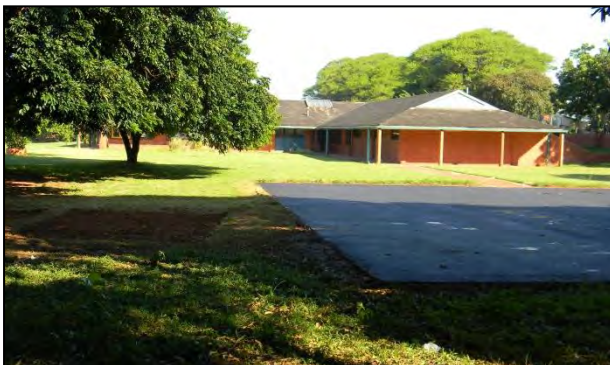
Figure 5.12 (Source: Author's Photograph, 2013) : View of facilities far from the community at Golden Hours.
