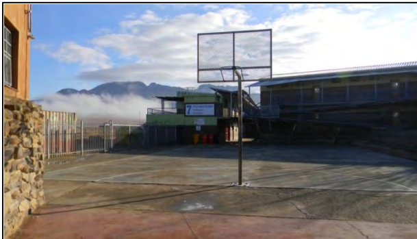
Figure 4.27 (Source: Author's Photograph, 2013) : Main courtyard overlooking community field and view.
