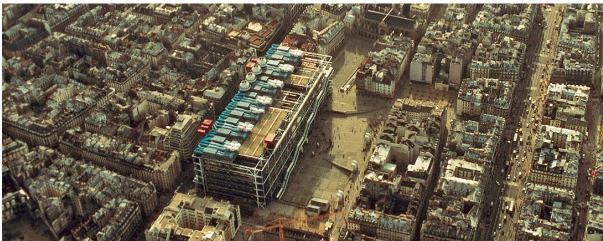
Figure 6: Aerial view of the Centre Pompidou (1977) (Source: http://www.richardrogers.co.uk )
