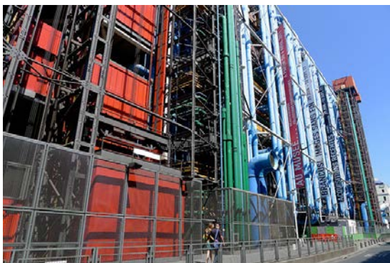
Figure 7: The Centres exposed service aesthetic (2011)
