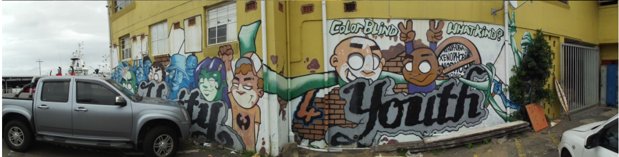
Figure 10: Graffiti Street Art on the external walls of the BAT Centre (2014) (Source: Author)
