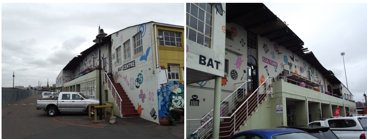
Figure 4 and 5: External view of the front façade of the BAT Centre (2014)
