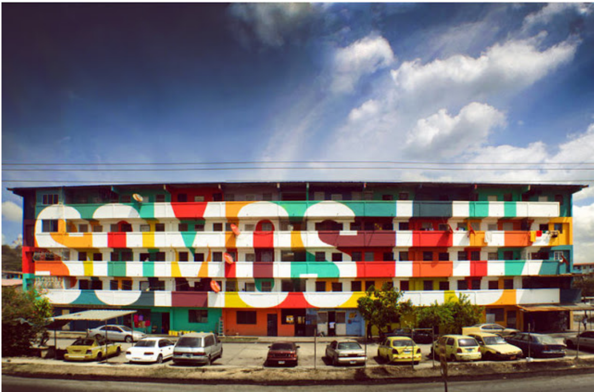
Figure 29: Revived concrete apartment block in Panama City by Boa Mistura (2013)
