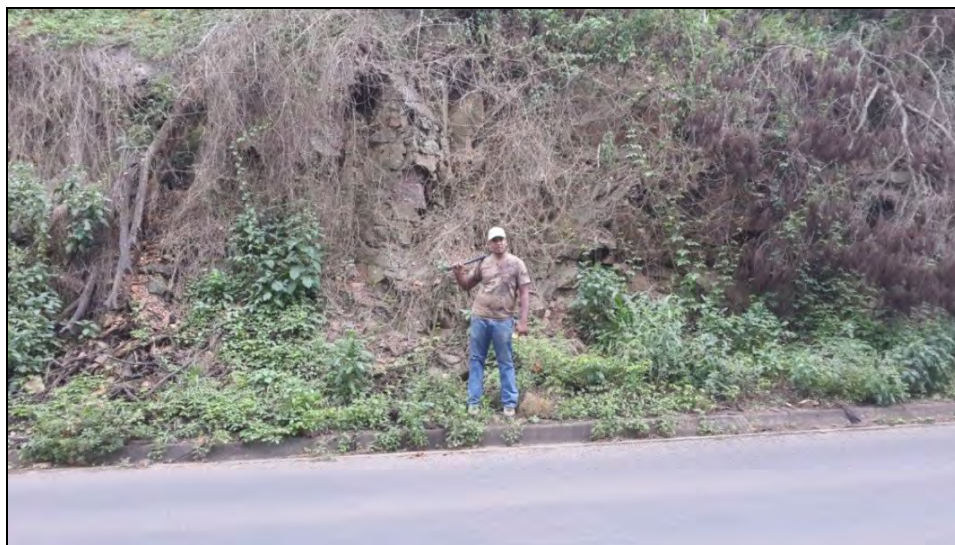
Figure 6.8: Exposure of the shale materials at Locality 4.
