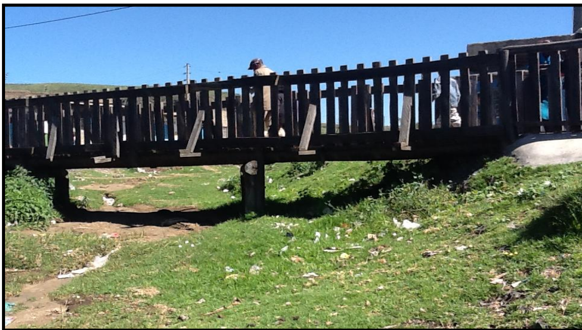
Figure 5: A poorly constructed CDF funded bridge in Longonot, Naivasha
