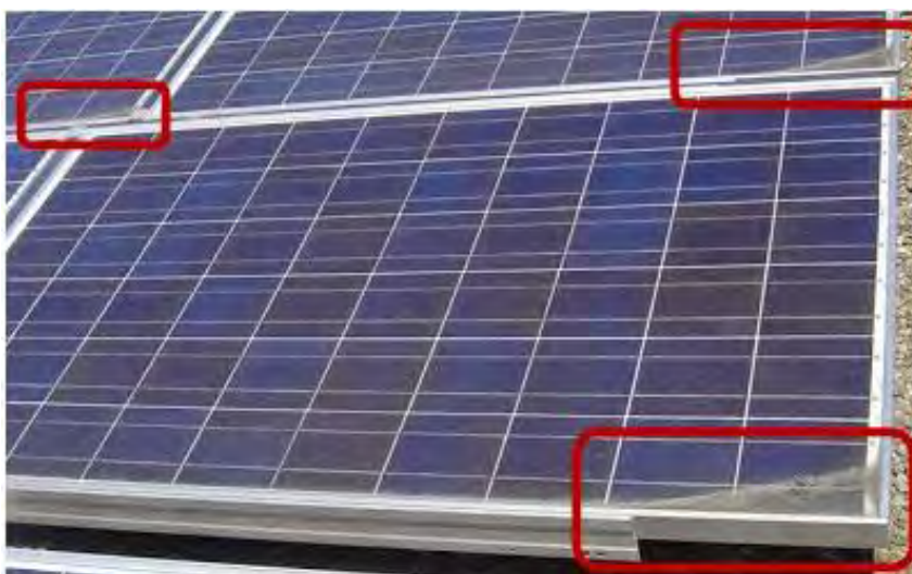
Figure 2-9: Accumulated dirt in the corners of a rooftop solar panel.
