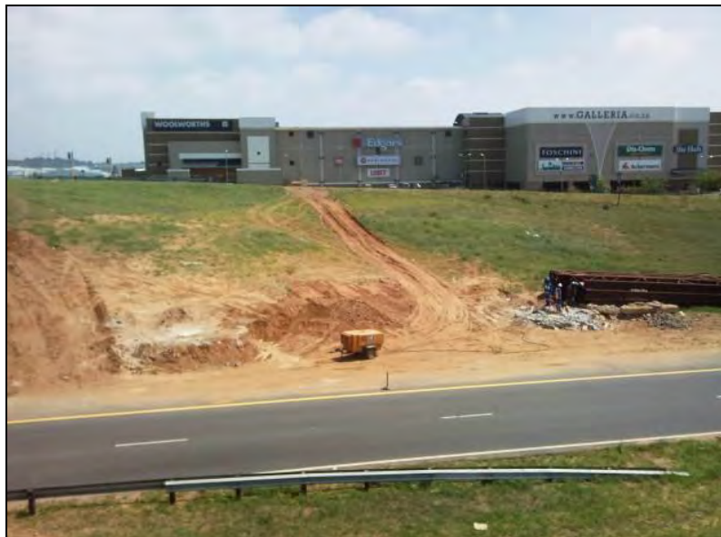
Plate 5.5 Ramp C embankment at Site Two in need of additional vegetation cover
