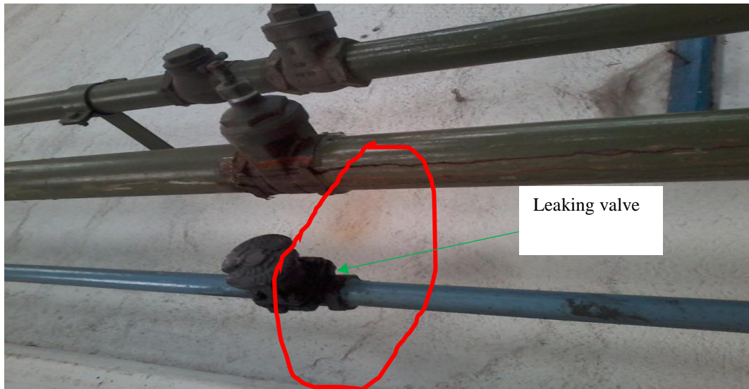
Figure 5-19: Leaking valve in the plant
