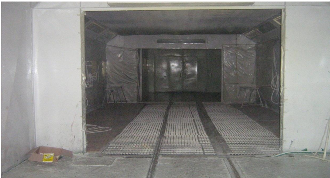
Figure 5-14: Front view of paint shop spraying booths
