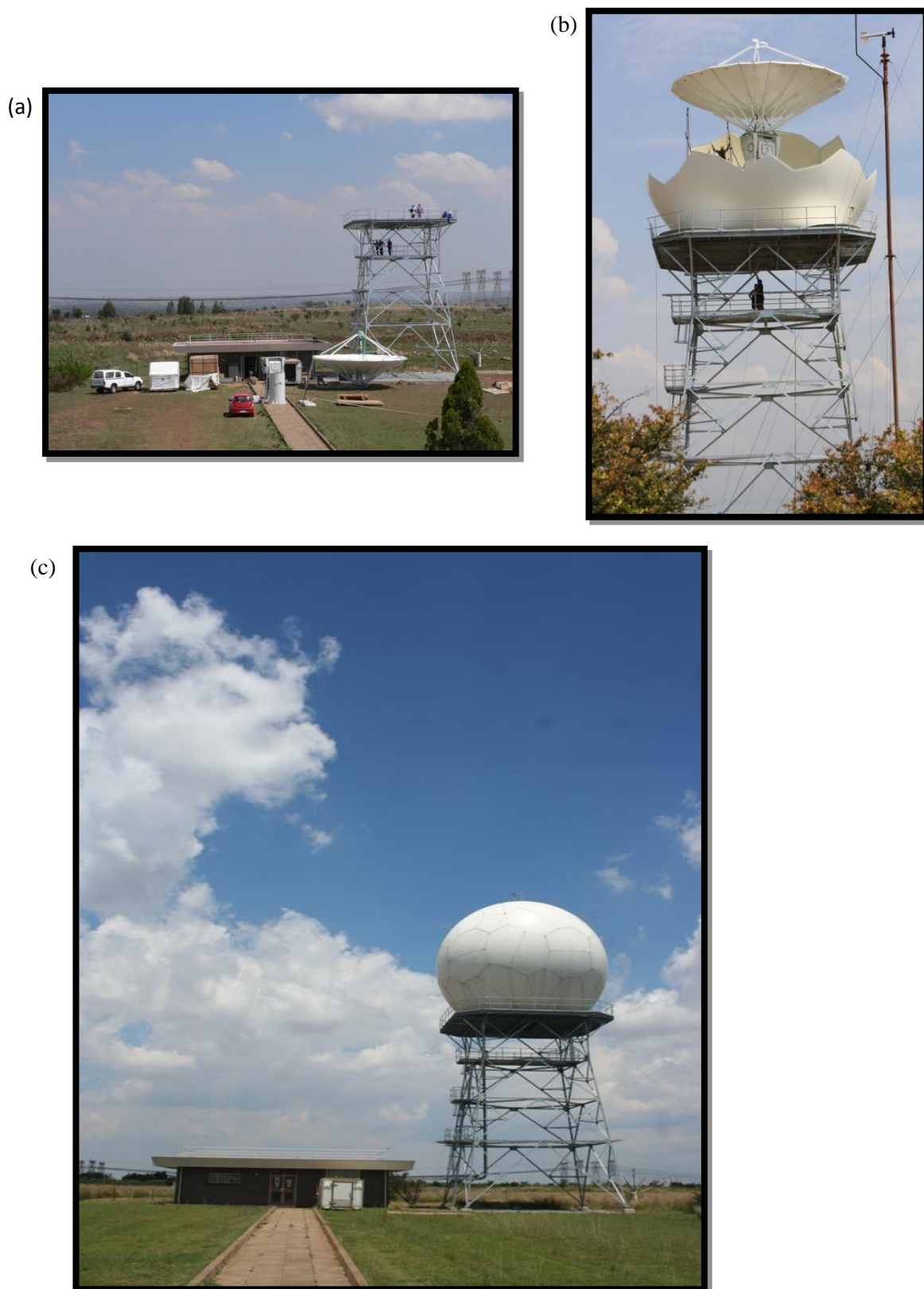
Figure 4-4: The Irene METEOR 600S S-band radar during construction in 2009, (a) and (b), as it stands today (c) at the Irene WO just outside Pretoria, Gauteng.
