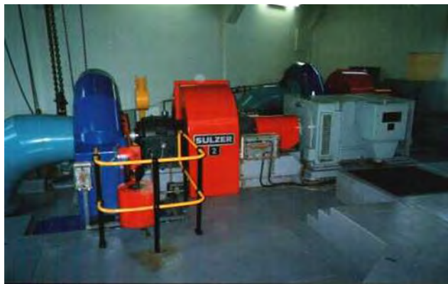
Figure 2.2: Small hydropower plant picture showing turbine and generator [36].
