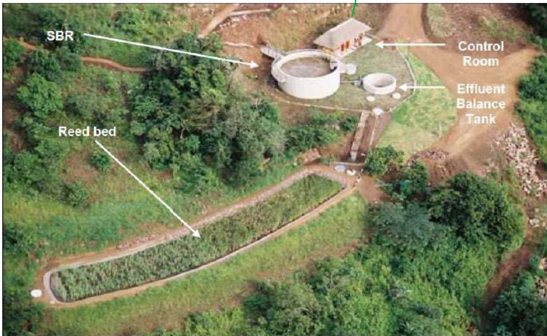
Figure 2-3 Aerial view of Mariannahill Leachate Plant (Sawyer, 2011)
