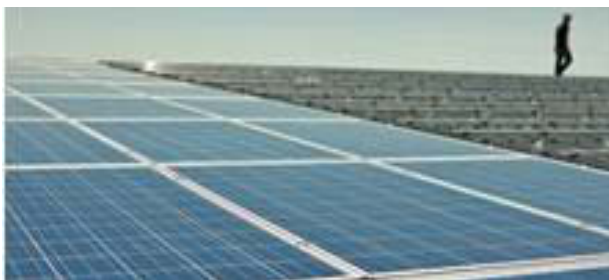
Figure 2-9 Photovoltaic Solar Panels (Dube Tradeport, 2014)
