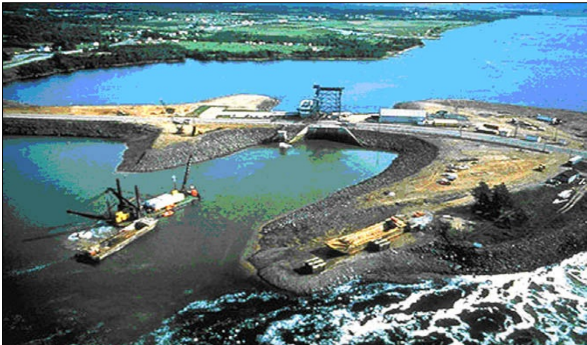
Figure 4-8: Annapolis tidal power facility, Rourke, et al. [43]
