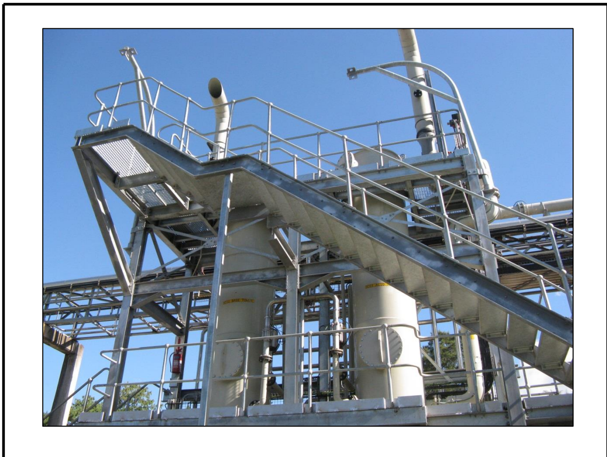
Figure 11: Company B's emission scrubbers
