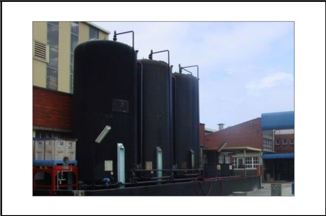
Figure 7: Company A's effluent tanks
