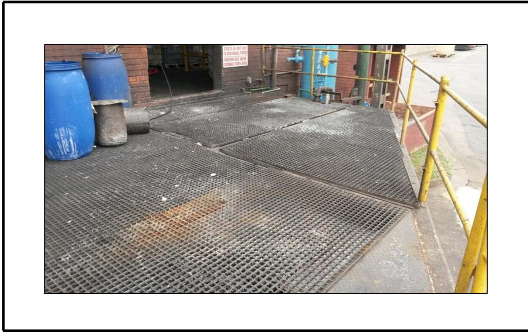
Figure 14: Top view of Company C's effluent tank which is located below the grid (the tank dimensions are 6m in length, 3m in width and 3 m in height)
