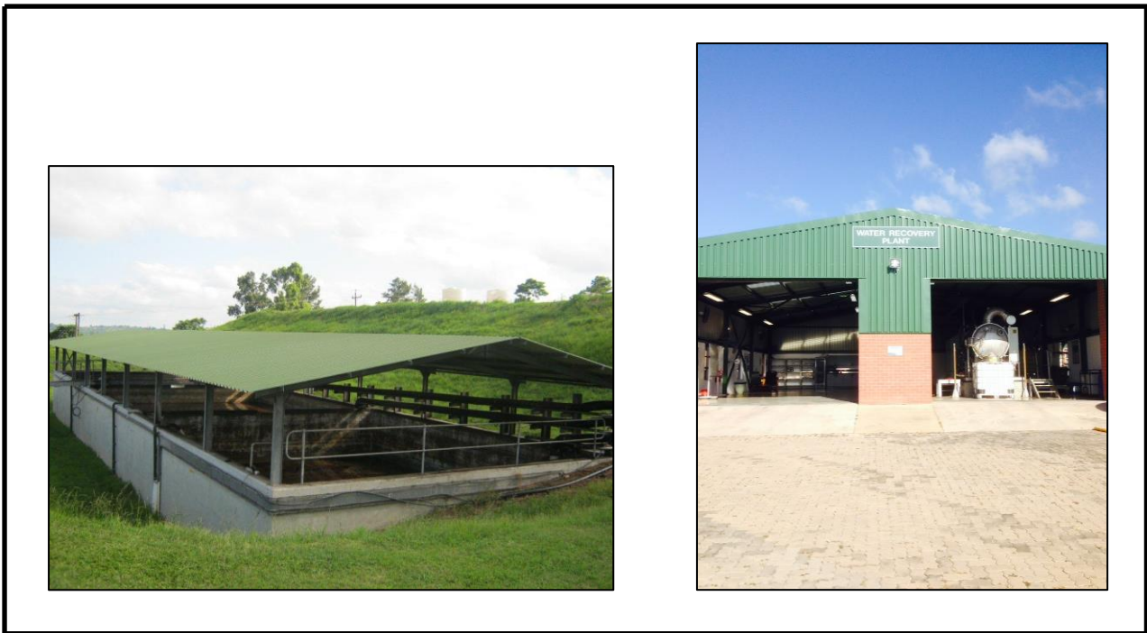
Figure 10: Company B's effluent pits and waste water recovery plant
