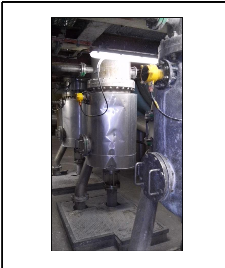
Figure 19: Company D's emission scrubbers
