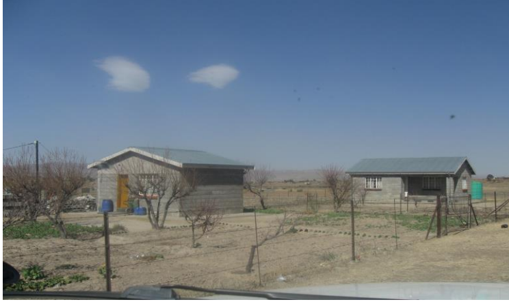
Figure 30 18 : Resettlement sample houses at Ha Makhalanya.
