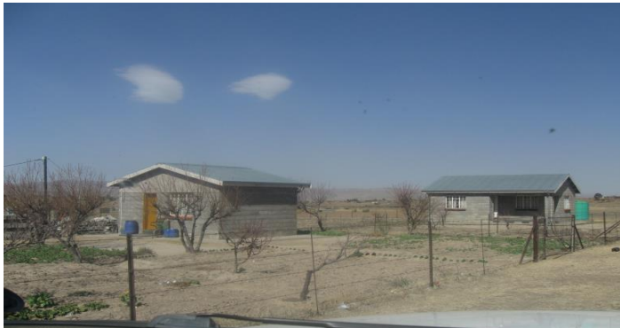
Figure 10: Example of Resettlement Houses
