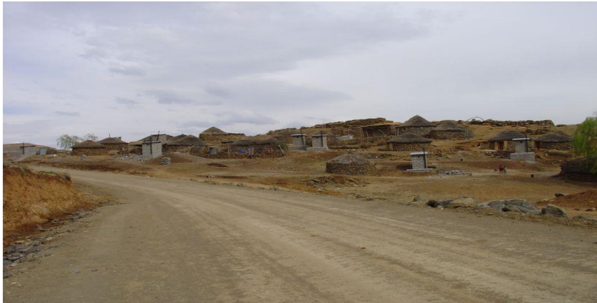
Figure 11: Improved latrines for disturbed communities
