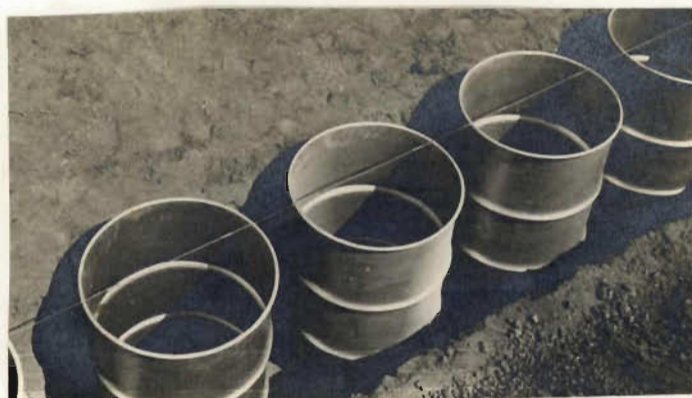
1a Pots lined up in trench prior to filling
