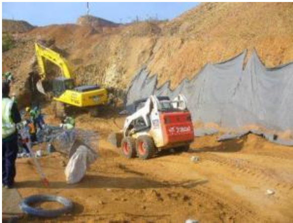
Figure 41: Excavator and skid-steer loader
