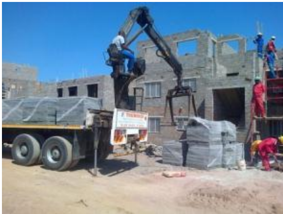
Figure 75: Crane operating truck
