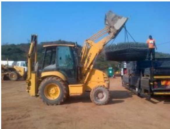
Figure 39: Tractor Loader Backhoe (TLB) near site office
