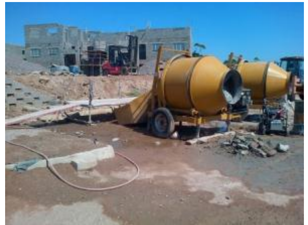
Figure 76: Concrete mixer and Fork lift
