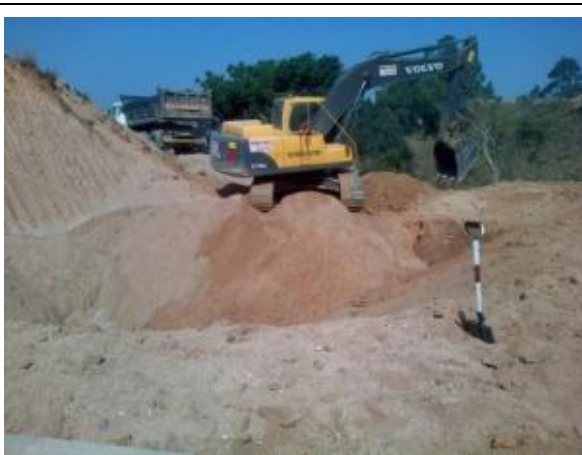
Figure 45: Truck and Excavator
