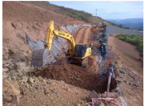
Figure 38: Excavator and Terramesh wall
