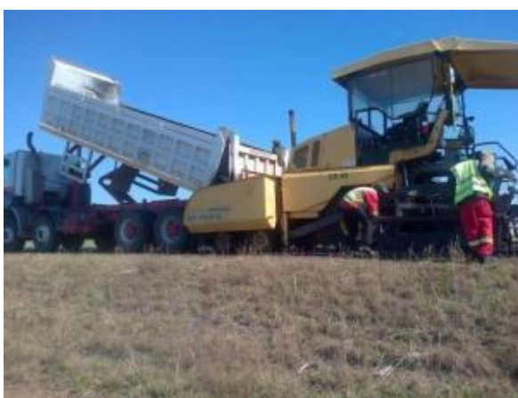
Figure 67: Truck and paver
