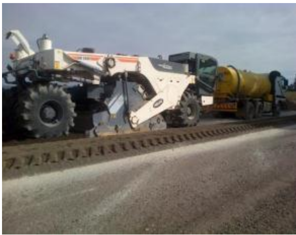
Figure 63: Cold Recycler and public road
