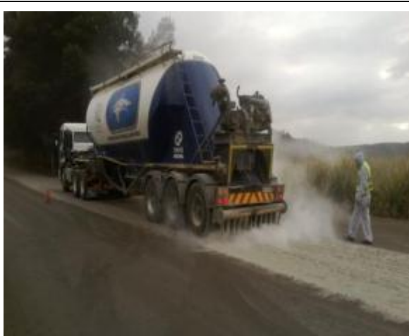
Figure 61: Truck cement spreader
