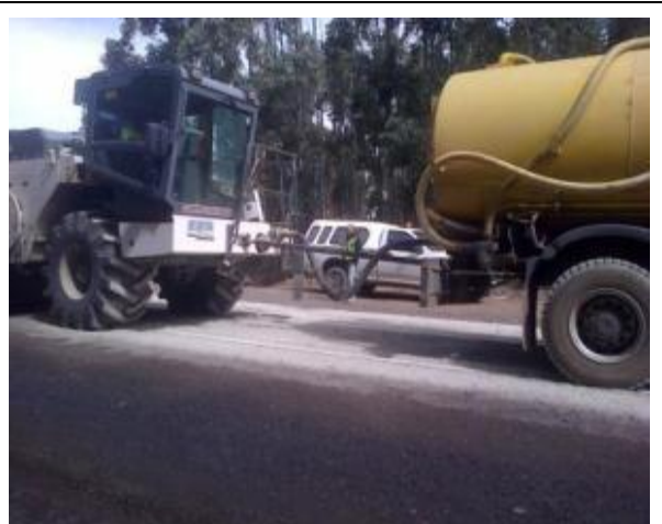
Figure 62: Cold Recycler and water cart
