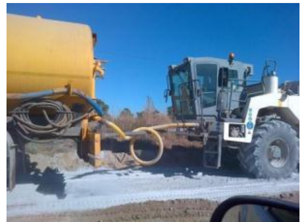
Figure 54: Water tack and recycler
