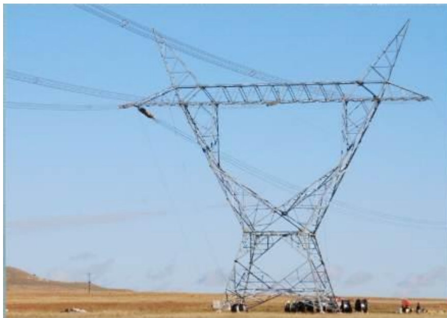
Figure 1-3: Example of Eskom Transmission lines 765kV Majuba-Umfolozi (South Africa)
