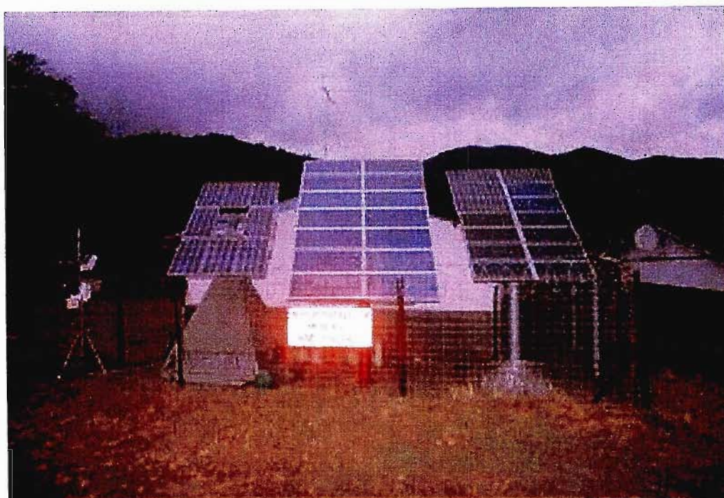
Figure 3.2: Solar/Gas Hybrid System at Myeka High School, 2000.
