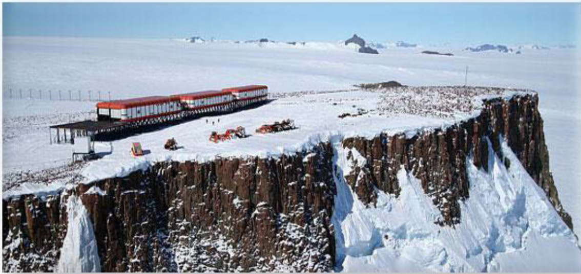
Plate 1: Outside view of SANAE station ( http://www.sanap.org.za ).
