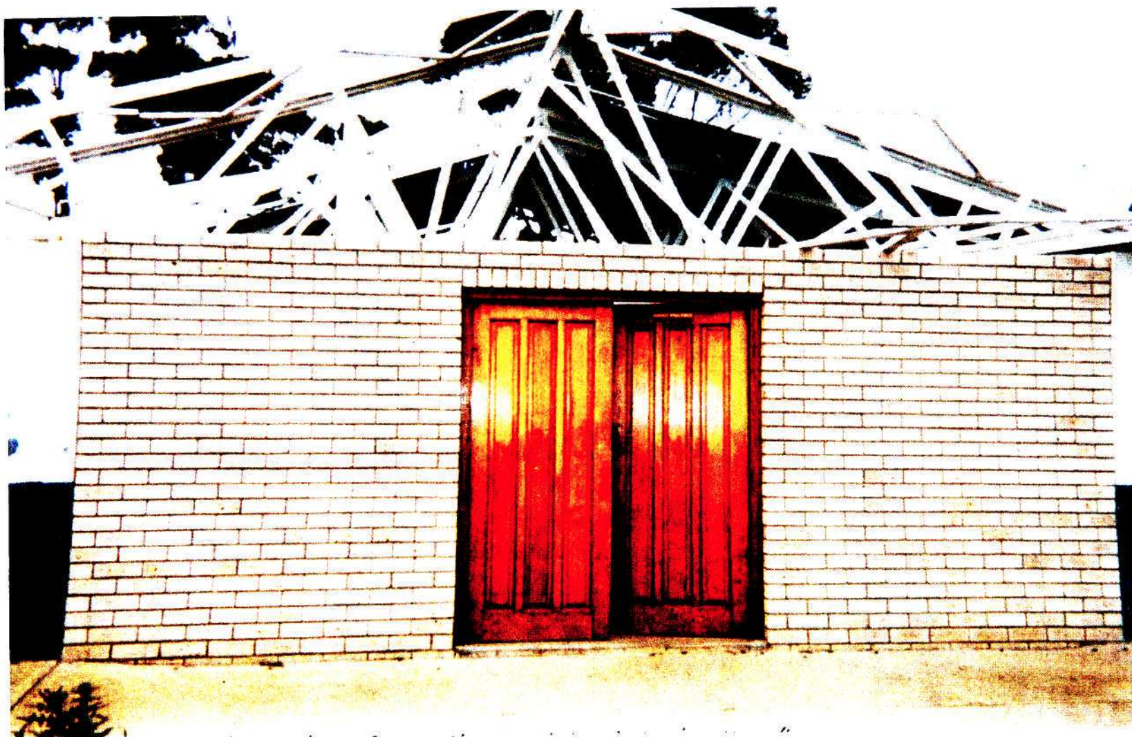
LIBRARY DAMAGED BY STORM, AT A NODAL POINT IN NKANDLA
