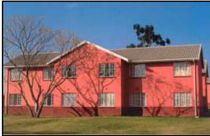
Figure 4.20 View of a typical block of apartments in Acacia
