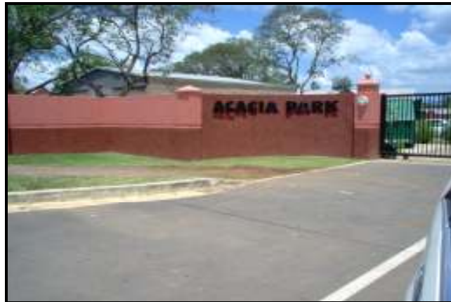
Figure 4.17 Main entrance of Acacia Park
