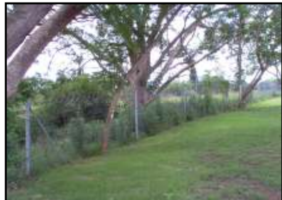
Figure 4.22 View of the perimeter fence.
