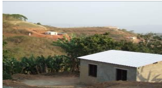
(Photograph 2): Complete Topstructure
