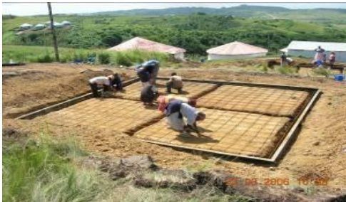
(Photograph 1): Casting of foundation/ slab
