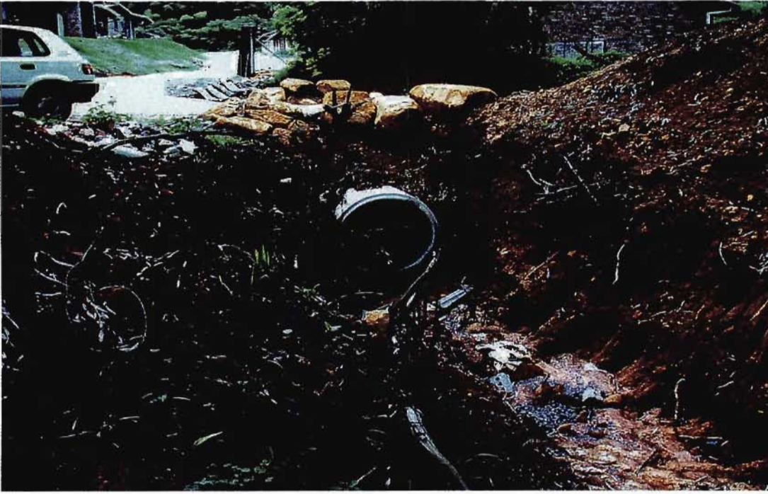
Plate 5.12 (c): Runoff from the swale is channelled through this pipe and into a detention basin. Note the erosion already taking place.
