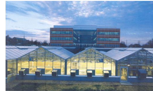
Illustration 4.3.1: The Danforth Centre treat the background with greenhouses facing the rear of the building (Mackeith 2002: 156).
