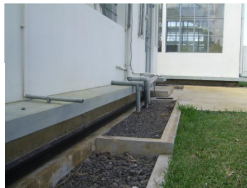
Illustration 7.15: Water surrounding the greenhouse to prevent any crawling insects from penetrating inside (Source: Author).
