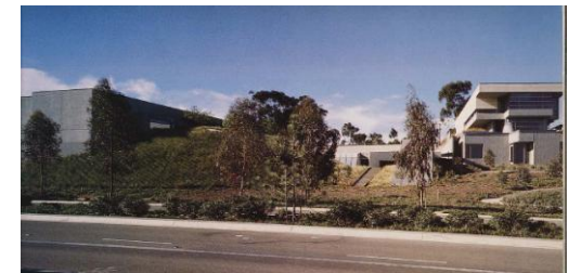
Illustration 4.4.3: The rear façade of the auditorium (left), the promenade from plaza (centre) and cantilevered theory centre (right); (Dietsch 1996: 89)
