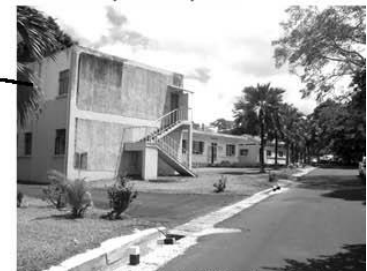
3. Two storey buildings for the MOA on Zoreil Road
