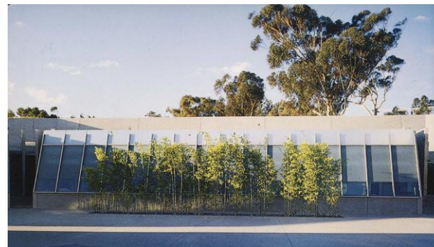
Illustration 4.4.9: The laboratory block's glazed panels, sandblasted on top, from parapet to rooftop terrace (Dietsch 1996: 86).
