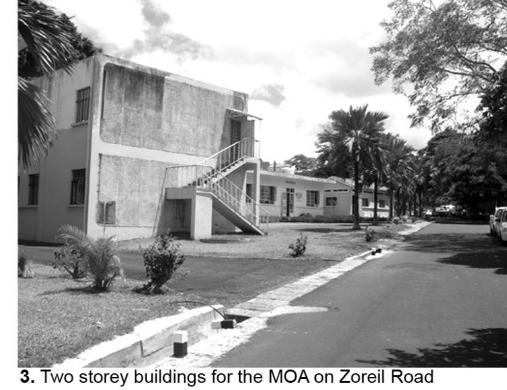
3. Two storey buildings for the MOA on Zoreil Road
