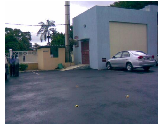
Illustration 5.2.3: Incinerator outside the building (Source: Author).
