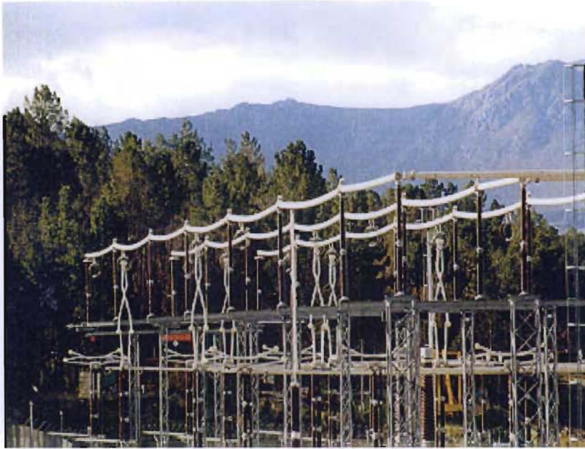
Figure 13.2: Unacceptable Vertical Deflection of a Tube Due to Own Weight
