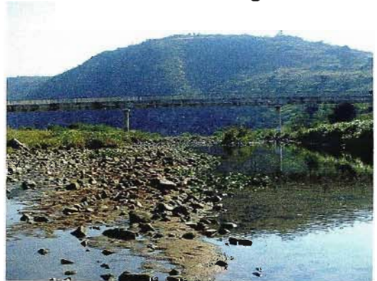
Umlazi J-Section Foot Bridge
