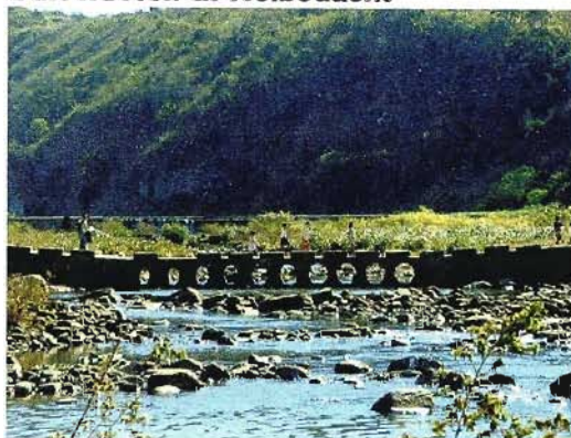
Culvert/Weir at Welbedacht
