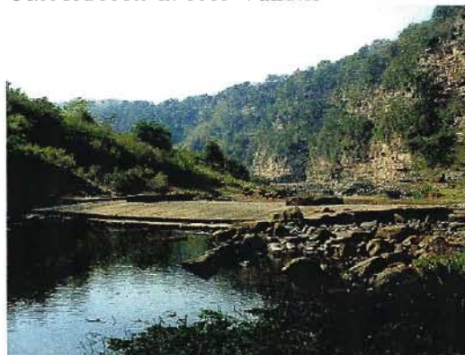
Culvert/Weir at Welbedacht
