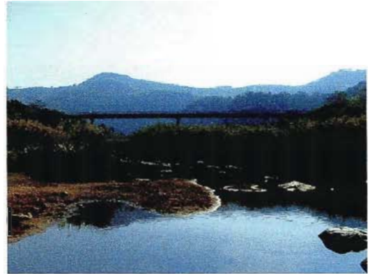
Umlazi H-Section Foot Bridge
