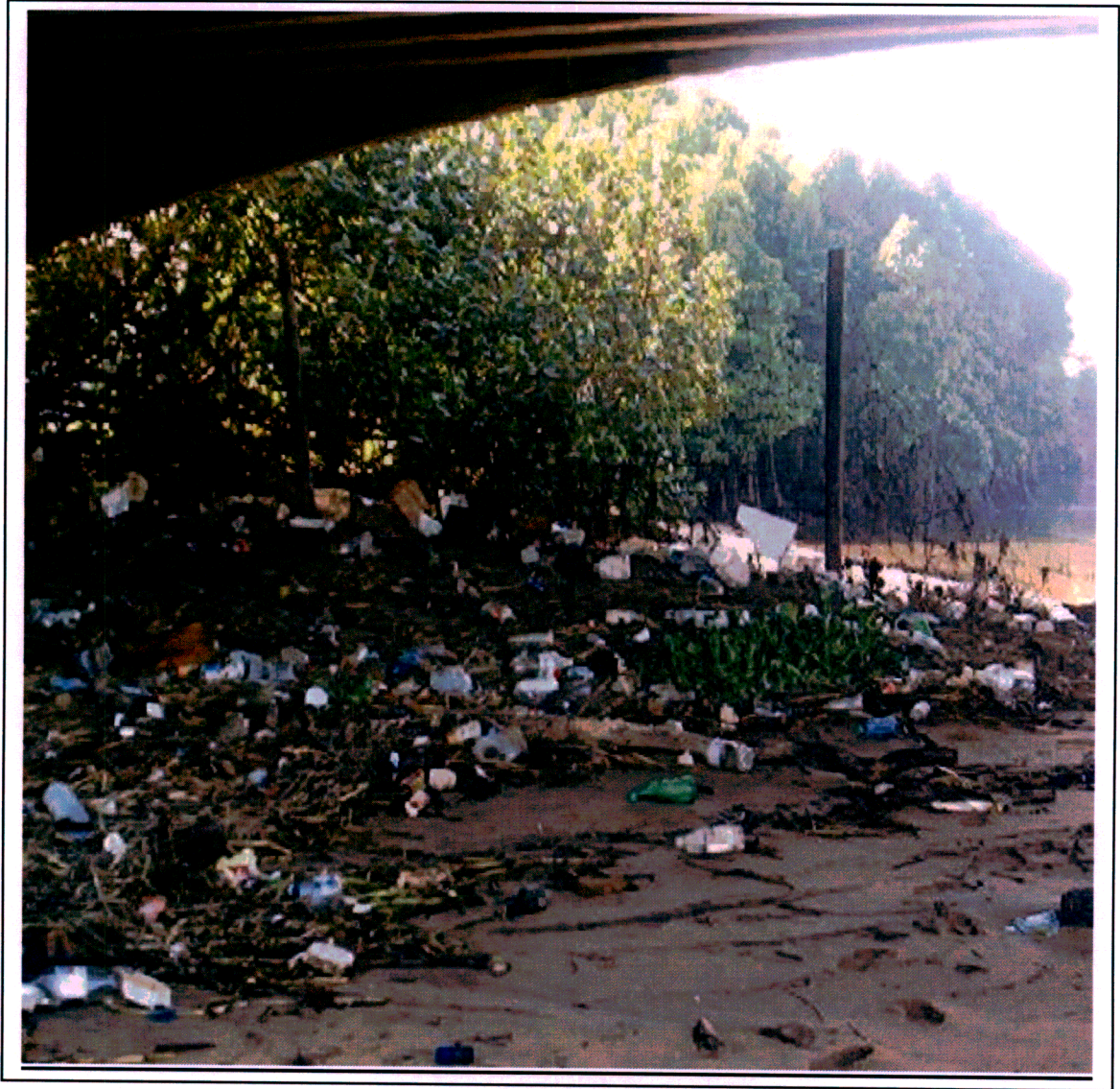
Plate 3.12 – Pollution found under the Ellis Brown Bridge. The sources of this pollution are from both vagrants that live under this bridge and from the pollution washed down by the tide.
