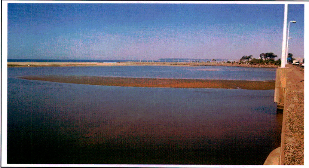
Plate 3.10 - A portion of the Mngeni Estuary from Ellis Brown Bridge to the mouth. Note that the outlet is secured on the south side by a solid groyne that penetrates into the surf zone. A 25m wide barrier bar separates the lagoon area visible above from the sea. Note also a large flood tidal delta in the central portion of the photo.
