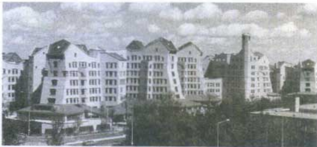
Fig. 6 Overall view of NMB Bank Headquarters (Vale & Vale 1991:54)
