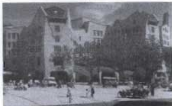
Fig. 10 The public square at the entrance (Vale & Vale 1991:53)
