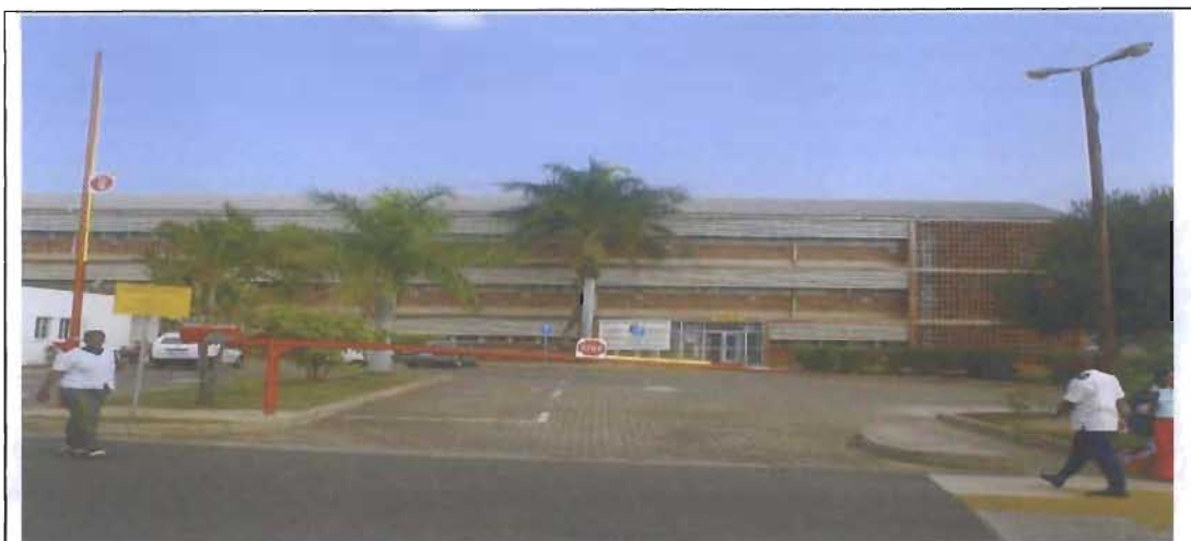
FIGURE 3.2 Photograph showing Ngwelezana hospital, Uthungulu Health District.
