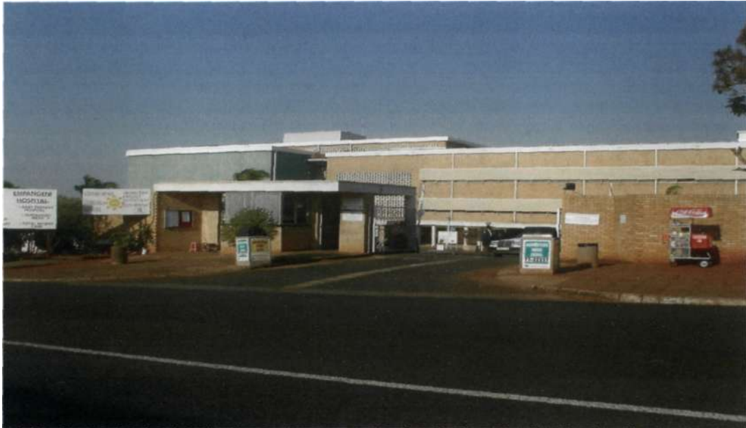
FIGURE 3.3 Photograph showing Lower Umfolozi District War Memorial hospital, Uthungulu health district.
