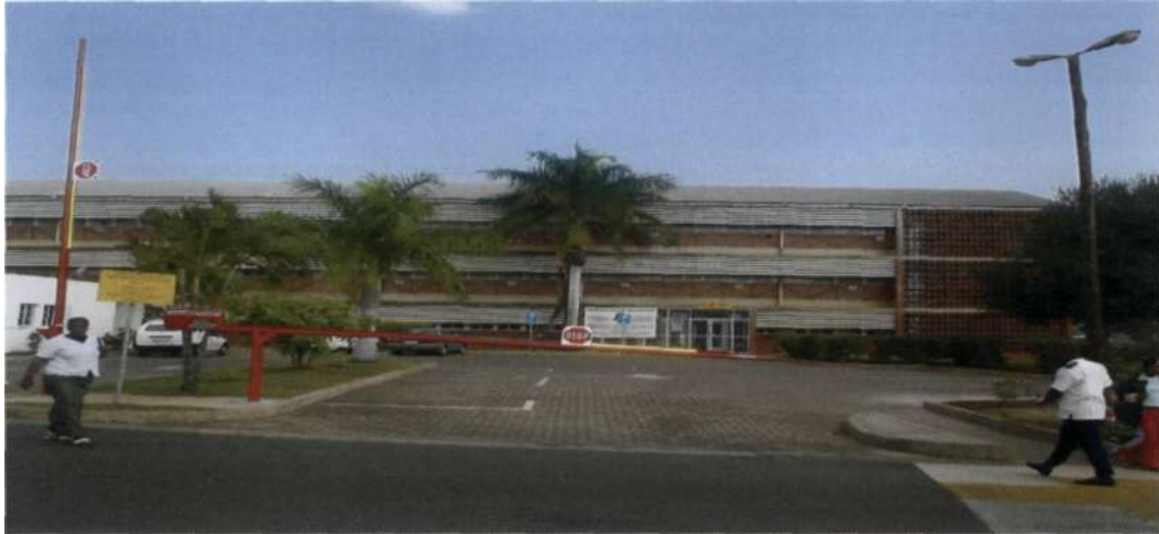
FIGURE 3.2 Photograph showing Ngwelezana hospital, Uthungulu Health District.
