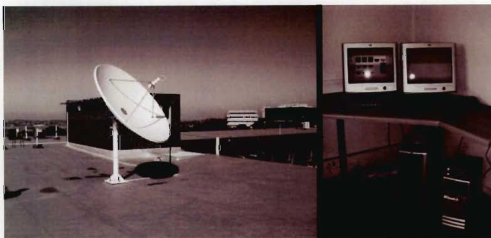
Fig. 3.12: Meteosat-8 C-band reception station and processing hardware at UKZN. The receiving PC and data processing server are shown.
