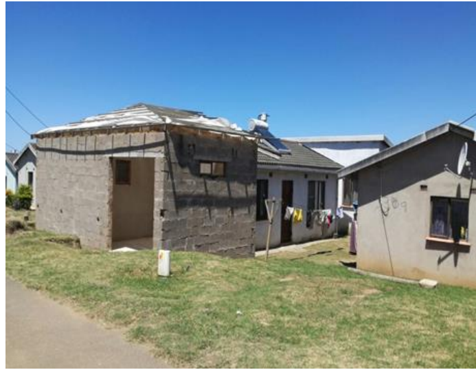
Plate 5.9 House extended too close to road because of the limited plot size
