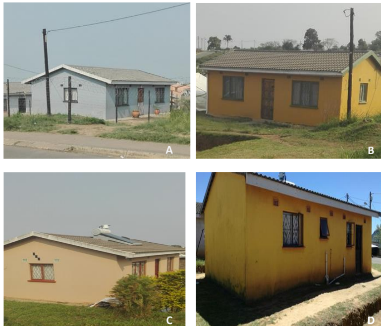
Plate 5.7 A, B, C. Examples of FEDUP housing units in Namibia Stop 8.
