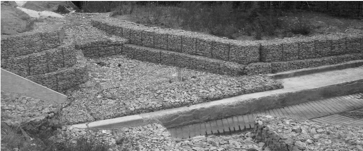
Figure 2.5: Typical Open-Air Stormwater Attenuation Pond in Johannesburg Area
