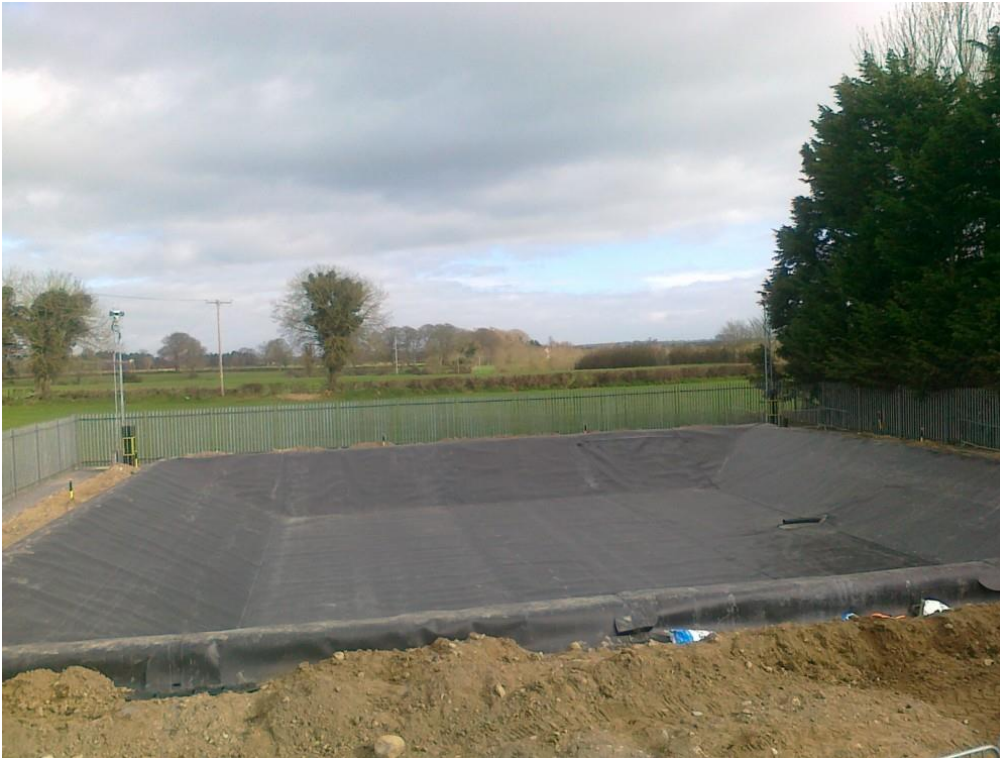
Figure 2.6: Construction of Attenuation Pond Using Geosynthetic Material
