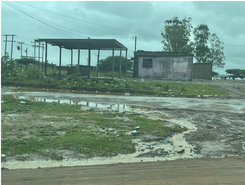
Figure 9: Access roads during rainy seasons
