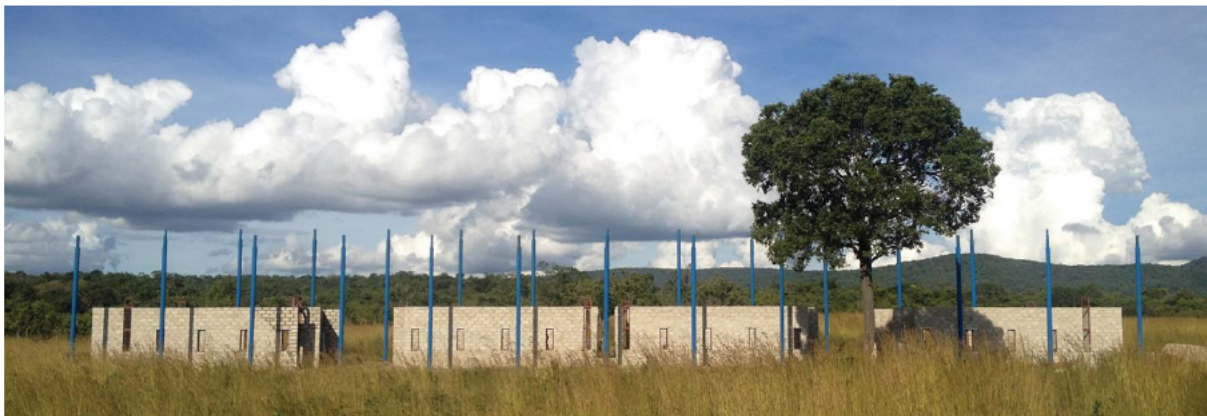
Figure 5.2.8 – Construction phase of school, Source: Archdaily, 2020
