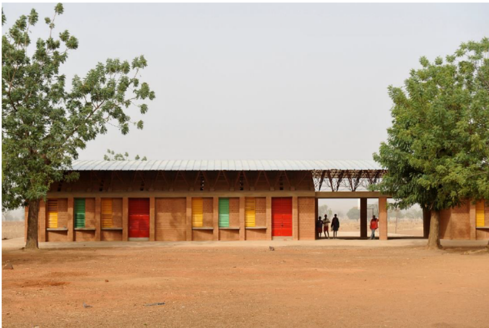
Figure 5.3.3 – Extension of Gando Primary School, Source: Archdaily, 2016
