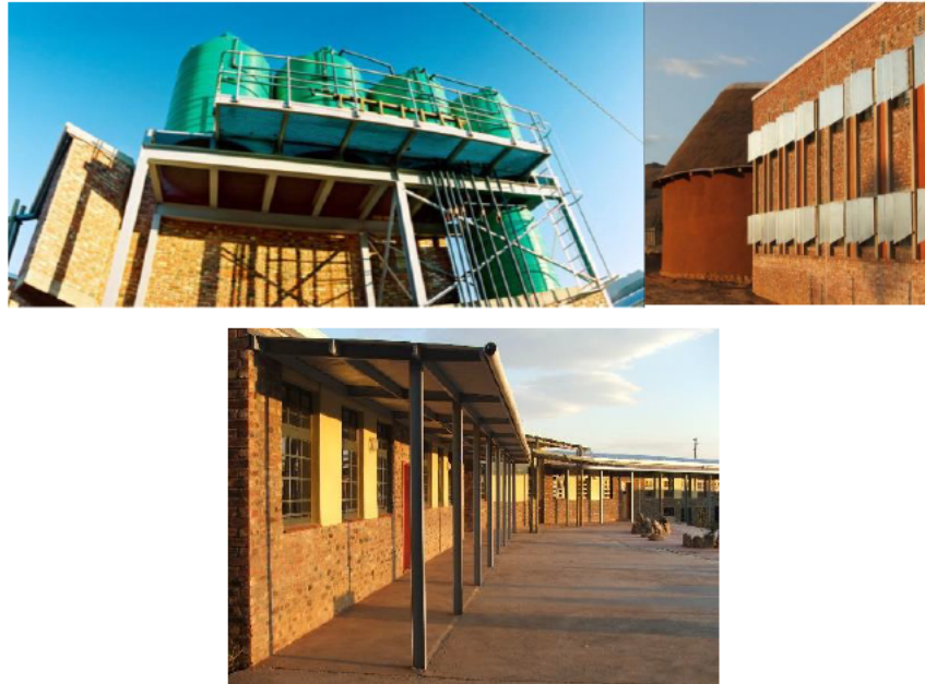
Figure 5.1.13 – Sustainable design strategies implemented in the school, Source: https://www.eastcoastarchitects.co.za , http://www.angelabucklandphotography.com
