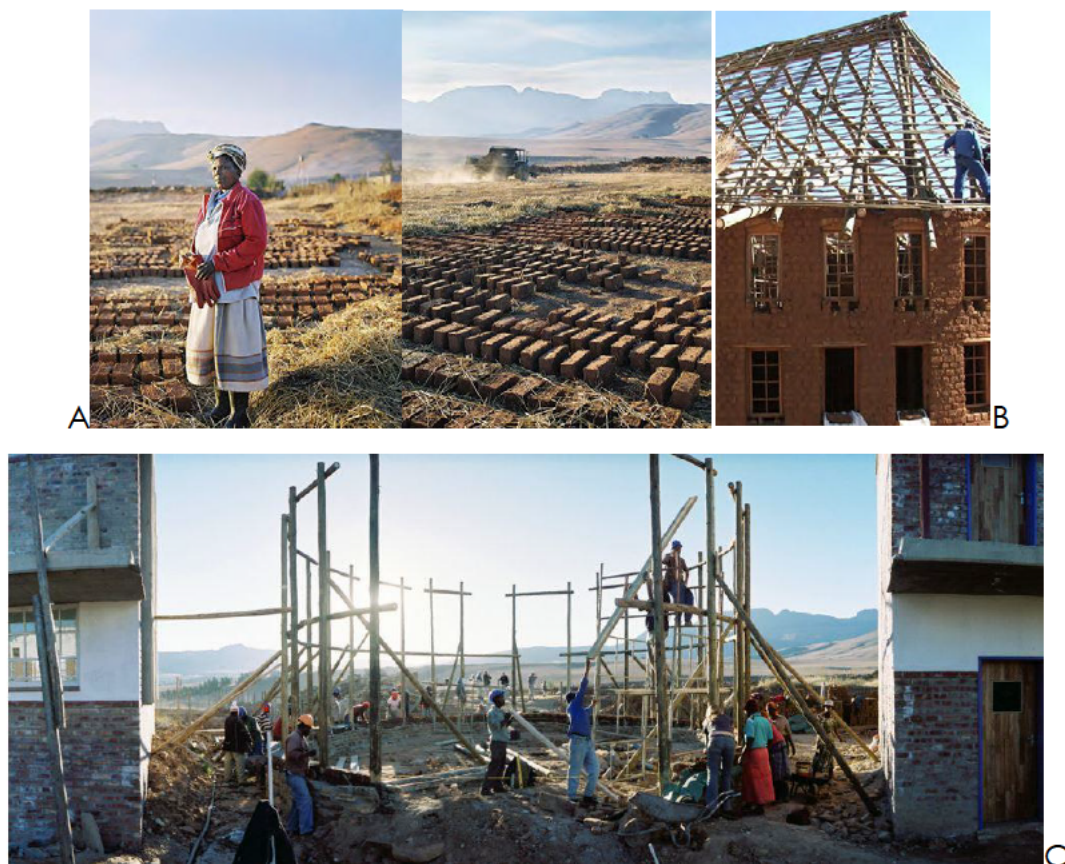
Figure 5.2.11 – (A) Woman making earth bricks, (B,C) Earth building under construction , Source: https://www.eastcoastarchitects.co.za , http://www.angelabucklandphotography.com
