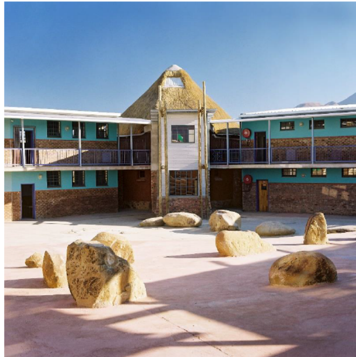
Figure 5.2.1 -View of the Seven Fountains Primary School, Source: https://www.eastcoastarchitects.co.za
