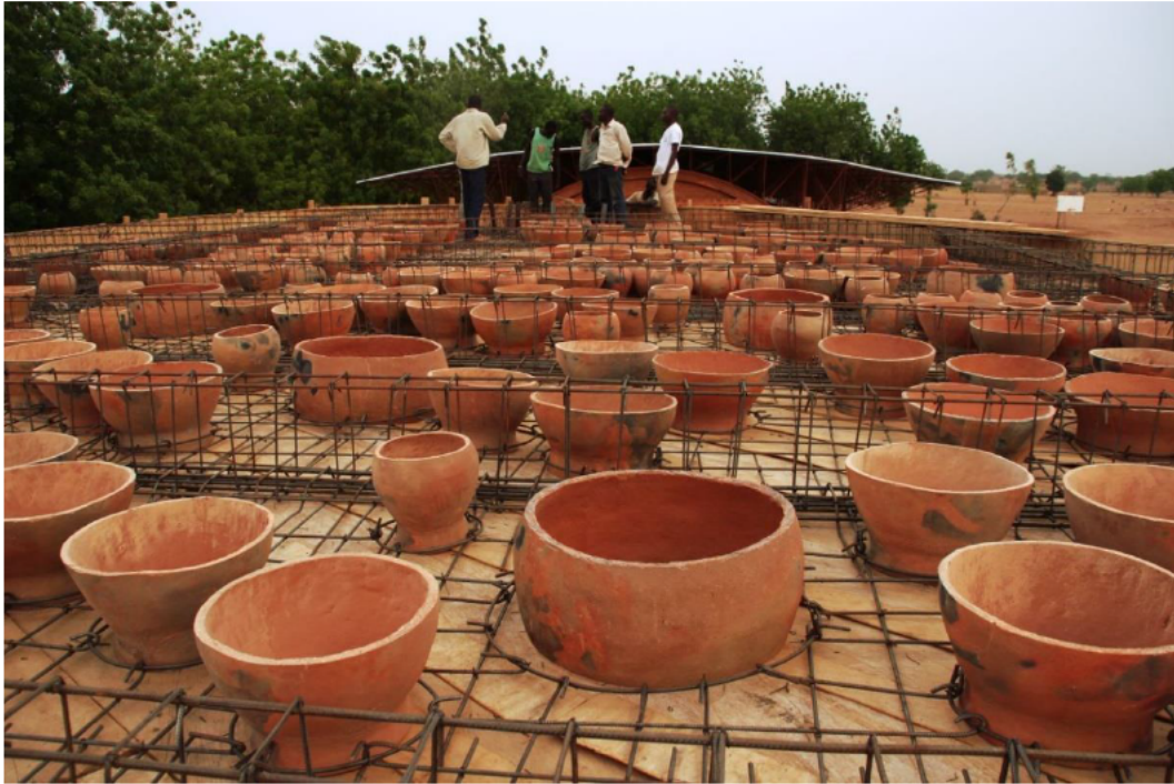
Figure 5.3.8 – Gando Primary School library roof construction , Source: https://images.adsttc.com/media/images/5024/1638/28ba/0d4e/9a00/00a2/slideshow/stringio.jpg?1414098347
