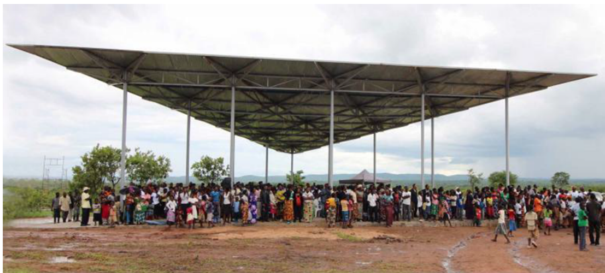
Figure 5.2.6 – Community gathering space, Source: https://www.world-architects.com , 2015
