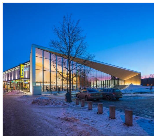
Figure 4.14 – Adjacent grocery store (K2S Architects, 2017)
