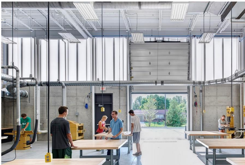
Figure 4.9 - Exposed building services in utilitarian vocational workshops (Neumann Monson Architects, 2017)
