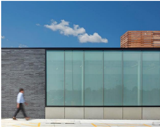
Figure 4.3 - Primary finishes (Neumann Monson Architects, 2017)
