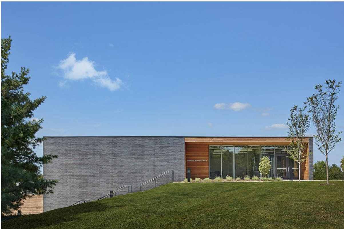
Figure 4.1 - South façade (Neumann Monson Architects, 2017)
