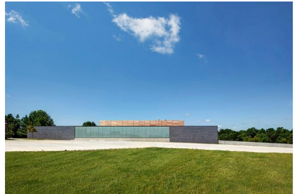
Figure 4.10 - East façade (Neumann Monson Architects, 2017)
