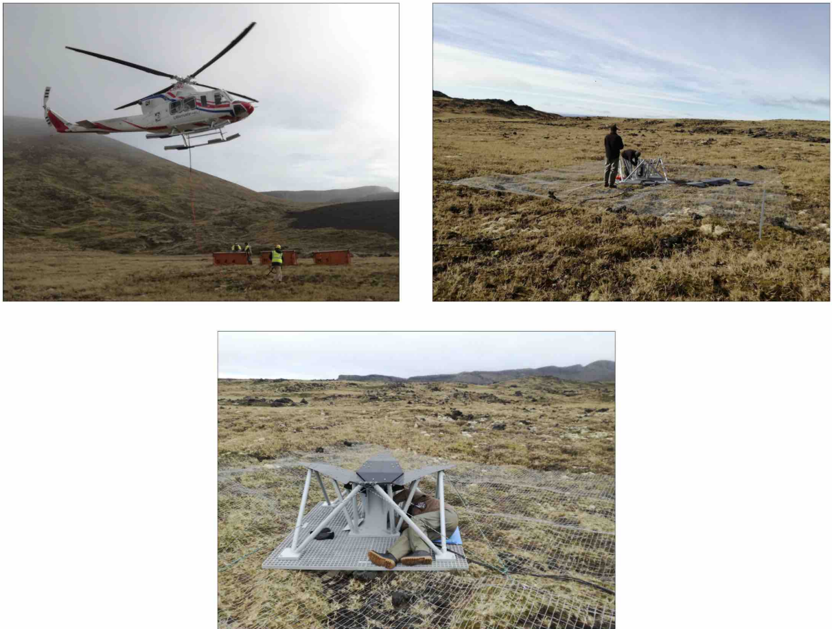
Figure 3.12: Clockwise from top-left : On-site cargo drop by the helicopter team; assembling the mechanical support structure; and installing the first stage module.
