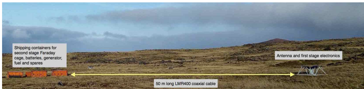
Figure 2.15: A wide angle view of a PRIZM antenna and shipping containers containing the second stage electronics, batteries, generator, fuel and spares. A 50 m long separation between the first and second stages help in minimizing self generated RFI.
