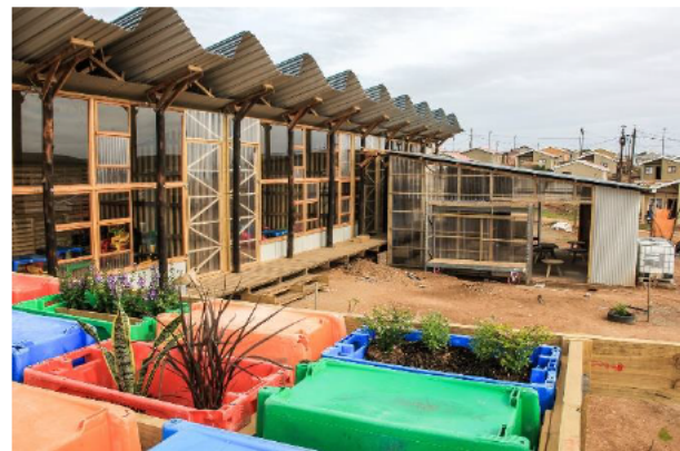
Figure 38: Silindokuhle Preschool. Source: https://www.designboom.com/architecture/collectif-saga-silindokulhe-preschool-joe-slovo-west-south-africa-07-28-2017/
