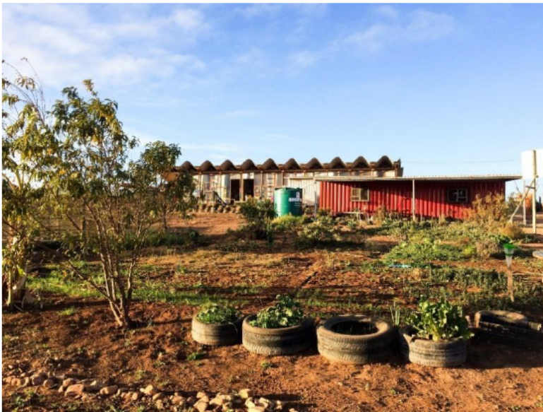
Figure 50: Surrounding Vegetation in Silindokuhle Preschool. Source: https://urbannext.net/silindokuhle-preschool/
