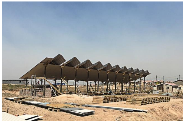
Figure 44: Roof Structure. Source: https://www.archdaily.com/875103/silindokuhle-preschool-collectif-saga
