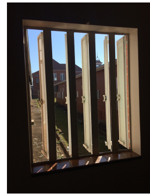
Fig.4.10. Impala Ward. - Corridor jail-like windows. Author's Own, 2016.
