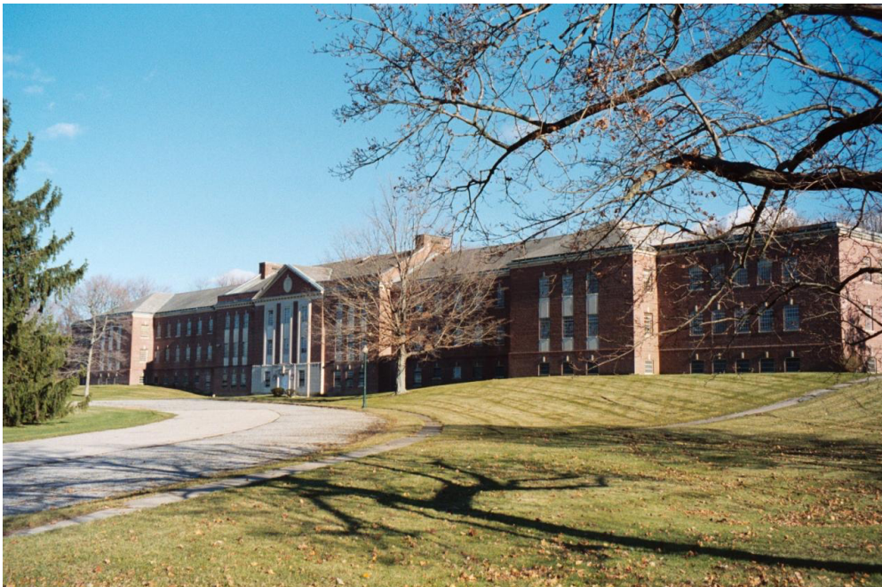
Fig. 3.19. Fairfield State Hospital. Abandoned Asylum, 2015.
