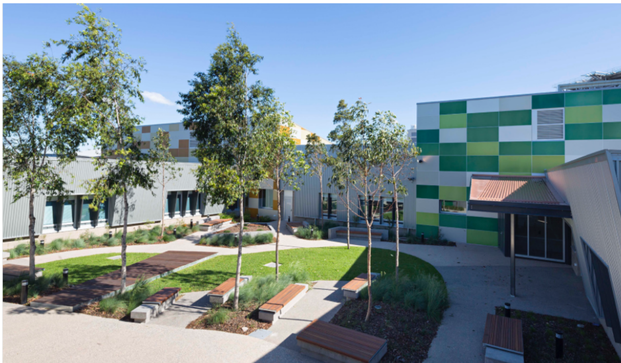
Fig. 6.6. Gold Coast University Hospital, Mental health Unit, Melbourne. Photograph by Christopher Frederick Jones. Hassel, 2014.
