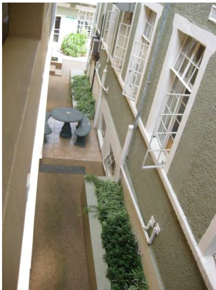
Figure 71: View Toward Paved Outdoor Seating Area between the Admin Extension and Original House (Author, 2013)
