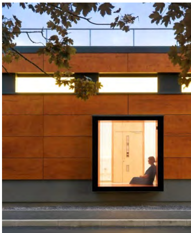
Figure 23: External View of Window Seat (source: www.fcbstudios.com )
