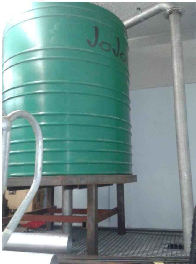
Figure 4.8: Supply tank with base to raise its level. The inlet pipe enters from the bottom and the discharge pipe enters from the top.
