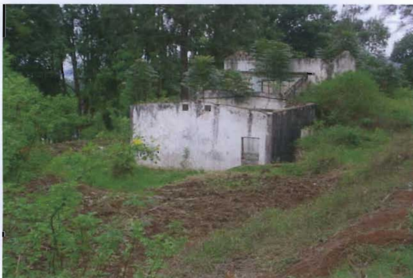
Plate 5.1. Residential buildings destroyed in Cyangugu town during the genocide
