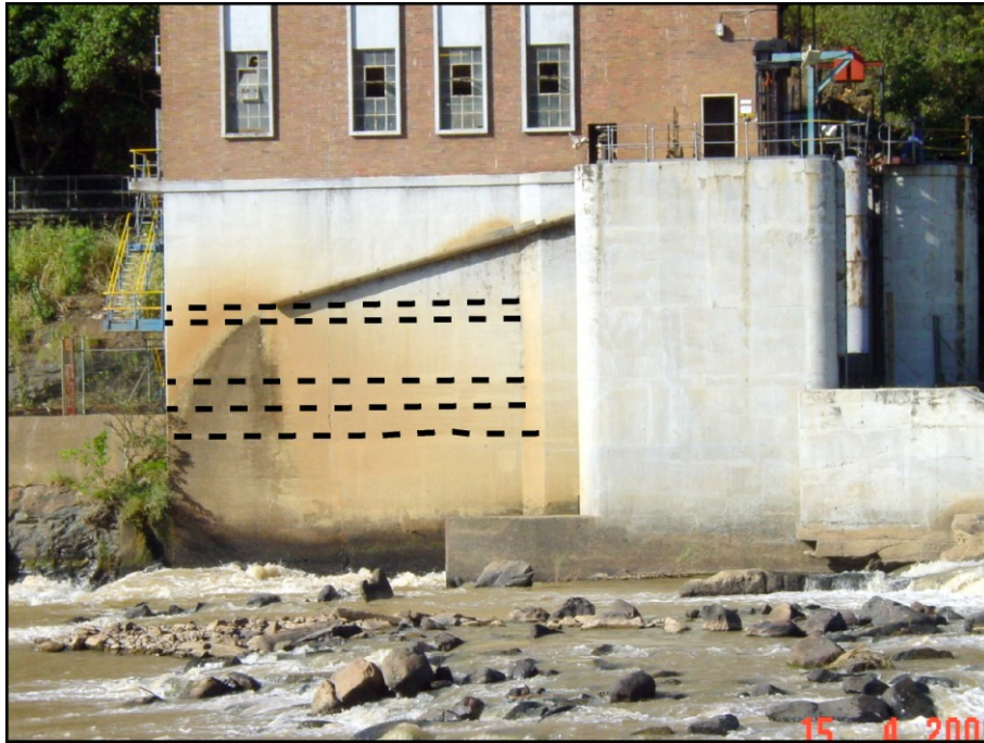
Figure 5.1. Photograph of flood marks on a pump station in the Mkomazi River. The dashed black lines indicate various flood elevations recorded on the pump station.
