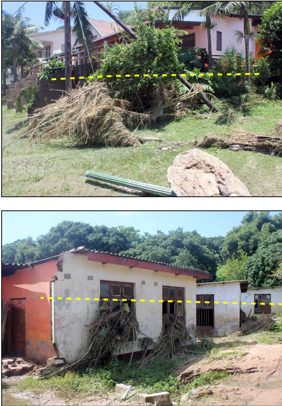
Figure 5.2. (Top) Accumulated debris along the Zotshe River. The dashed yellow line indicates a flood elevation from 2012. Floods in 2009 covered the roof of the house. (Bottom). A flood damaged house along a tributary of the Mzinto River in 2012. The yellow dashed line represents the flood elevation.
