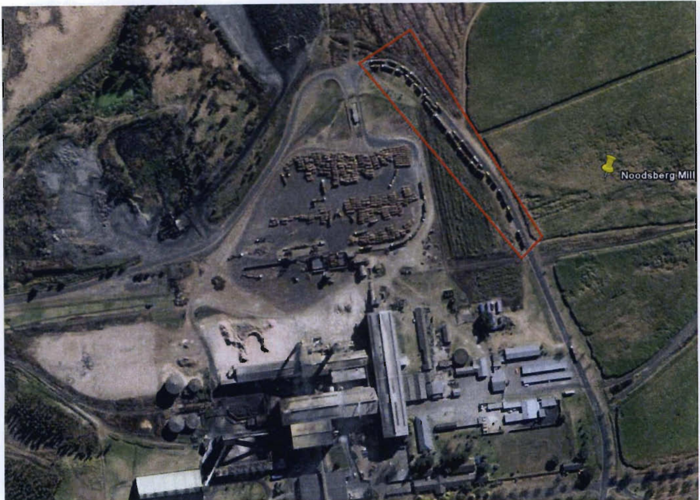
Figure 4.10: Google Earth Satellite image of the Noodsberg Mill area - Rectangular box highlights extreme queues outside mill-yard
